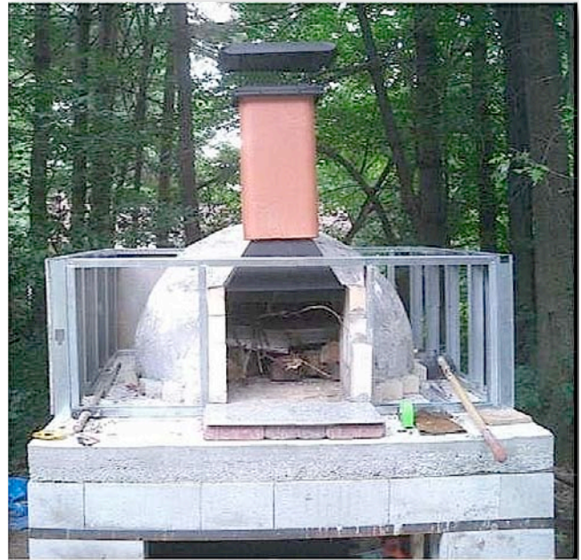
10.2. The vent attached to a terracotta chimney and fully enclosed.
