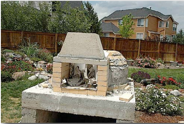
10.7. The cast vent set in place with brick vent walls.
