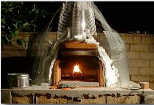
15.4 Rebar and lathe shape the Igloo.
