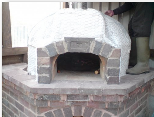
13.2 Multiple layers of FB Blanket.
