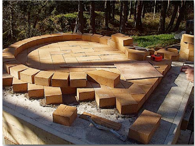
5.6. The cooking floor with the first course laid out.
