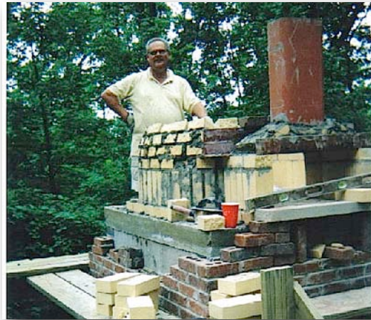
12.1. Refractory flue liner.
