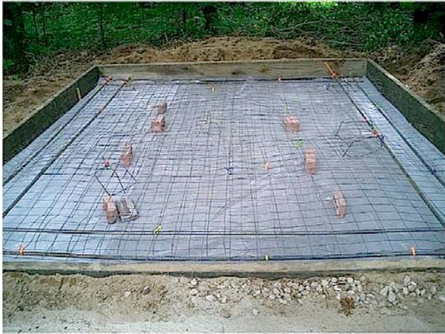
1.3. Framed, lined, with wire mesh and rebar.
