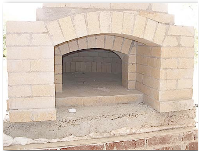
11.3. Different style brick arch with setback.
