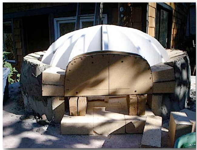
8.4. A form shapes oven opening.
