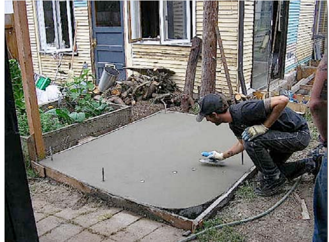
1.5 The finished foundation ready to cure.
