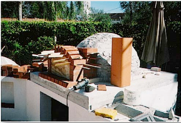
11.1. A decorative brick arch forms the vent opening.
