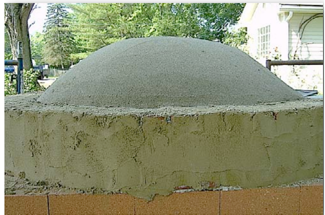
6.4 Sand form inside first course for bricks.
