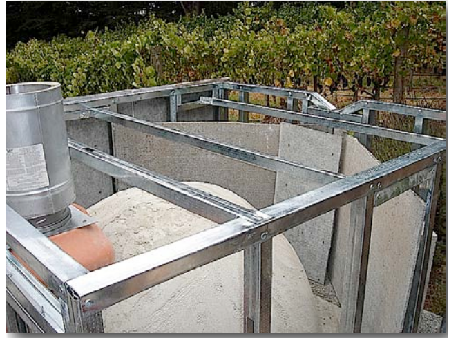
13.5 Concrete board blocks off the corners.
