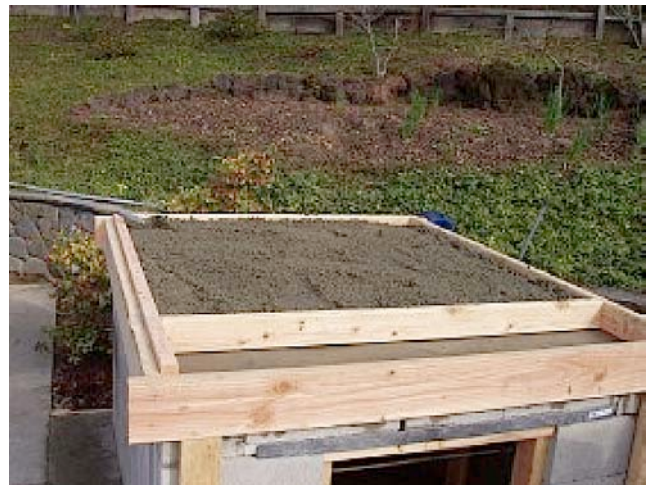
4.6. Vermiculite concrete poured under the oven chamber.
