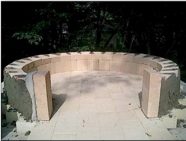
7.1. First course a half brick set upright.
