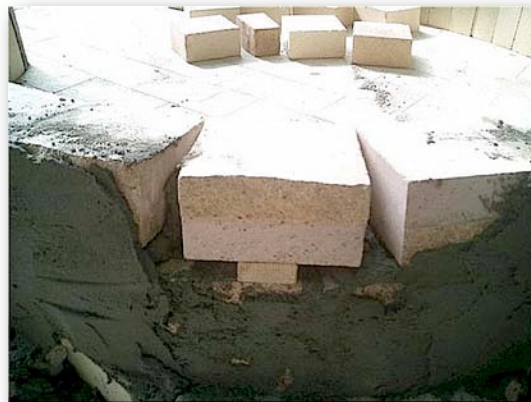
7.5. Using a shim to shape the dome without forms.
