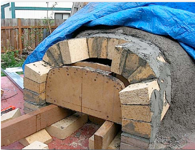
10.4 Another brick vent.
