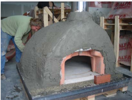
15.5 Rough coat of stucco on wire lathe.
