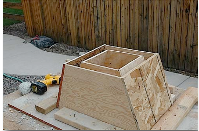
10.5. Construct the form using plywood.
