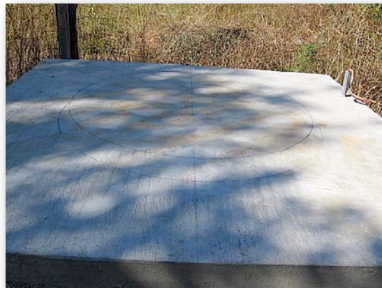
5.3 Measure carefully where the oven will sit.
