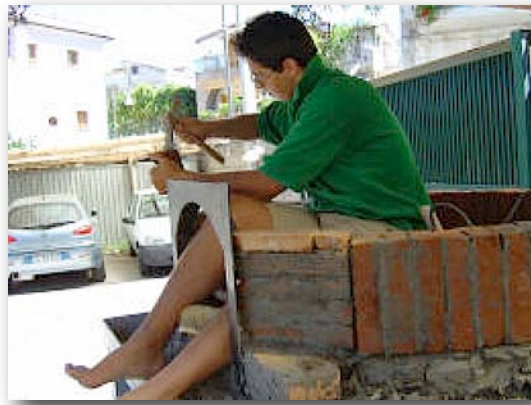
7.3. A full height brick upright in the first course.
