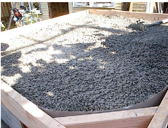
4.5. Insulating concrete on top ready to cure.
