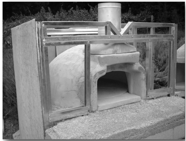
16.5 Metal studs walls with a shed roof.
