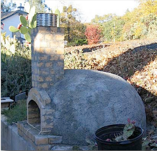
15.3. The oven dome and lathe shape the Igloo.
