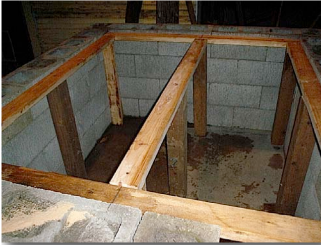
3.1. The form support ready for the tray.
