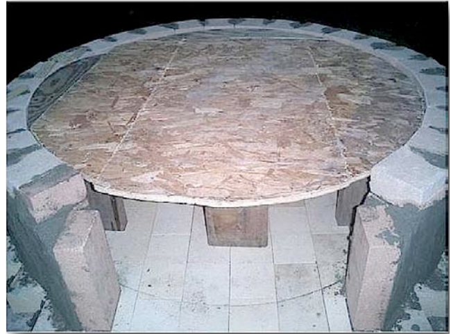
9.1 A removable form inside the oven.
