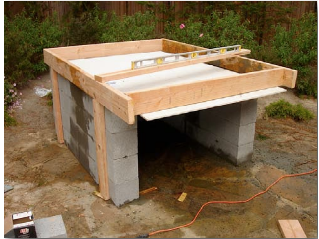
3.3. Hardibacker inside the side forms.
