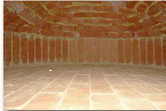
A taller first course and steeper, lower dome characterize the Naples-style oven.
