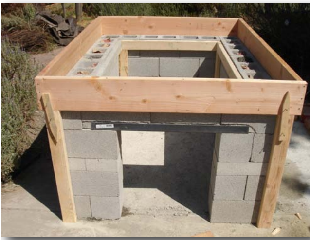
3.5 Form sides held in place with 2"x4"s.
